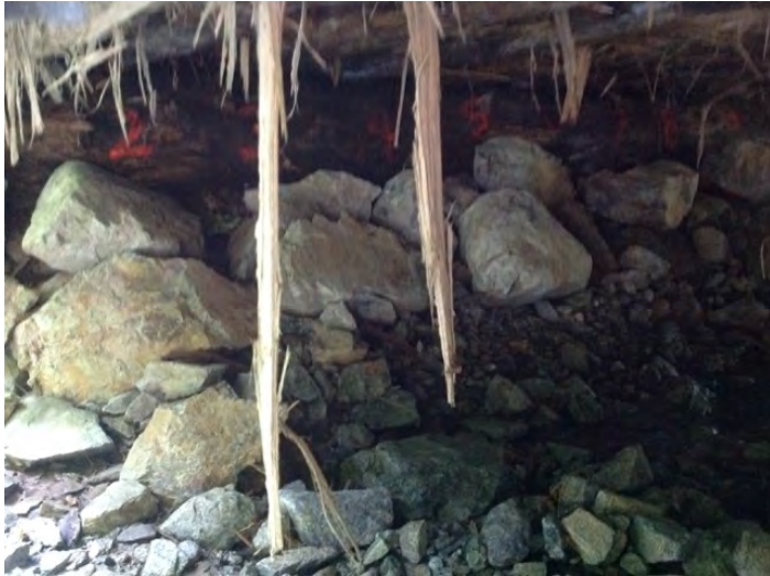
Left Bank Abutment when facing downstream
