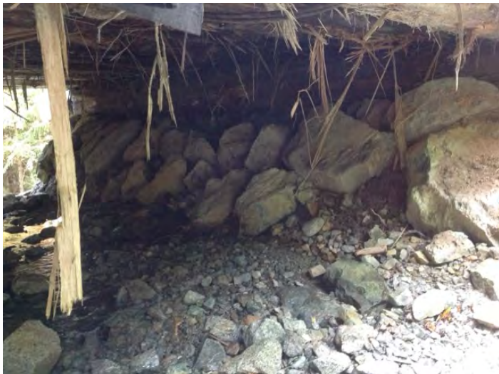
Right Bank Abutment when facing downstream
